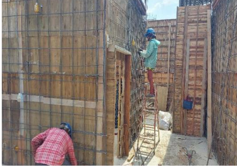
C棟B1F牆筋綁紮 宏峻6/20
