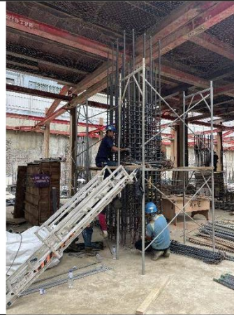
BC棟 B2FL柱筋綁紮 宏峻5/8
