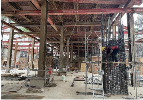
BC棟 B2FL柱筋綁紮 宏峻5/8
