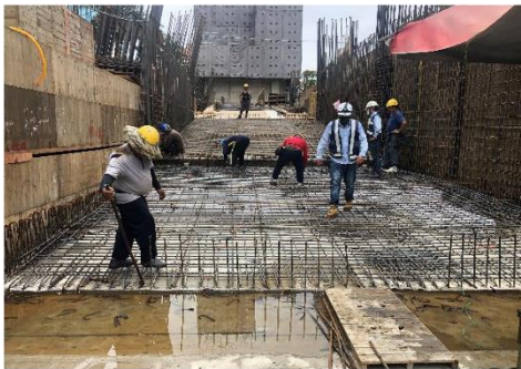
A區車道版鋼筋綁紮 宏峻6/23
